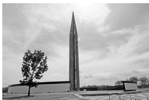
Capas Memorial: The large scale of the monument is quite proportional to the vastness of its setting
